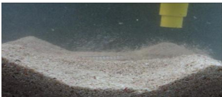
(g) A few more passes are made over the pipeline using the Mass Flow Excavator (MFE).
